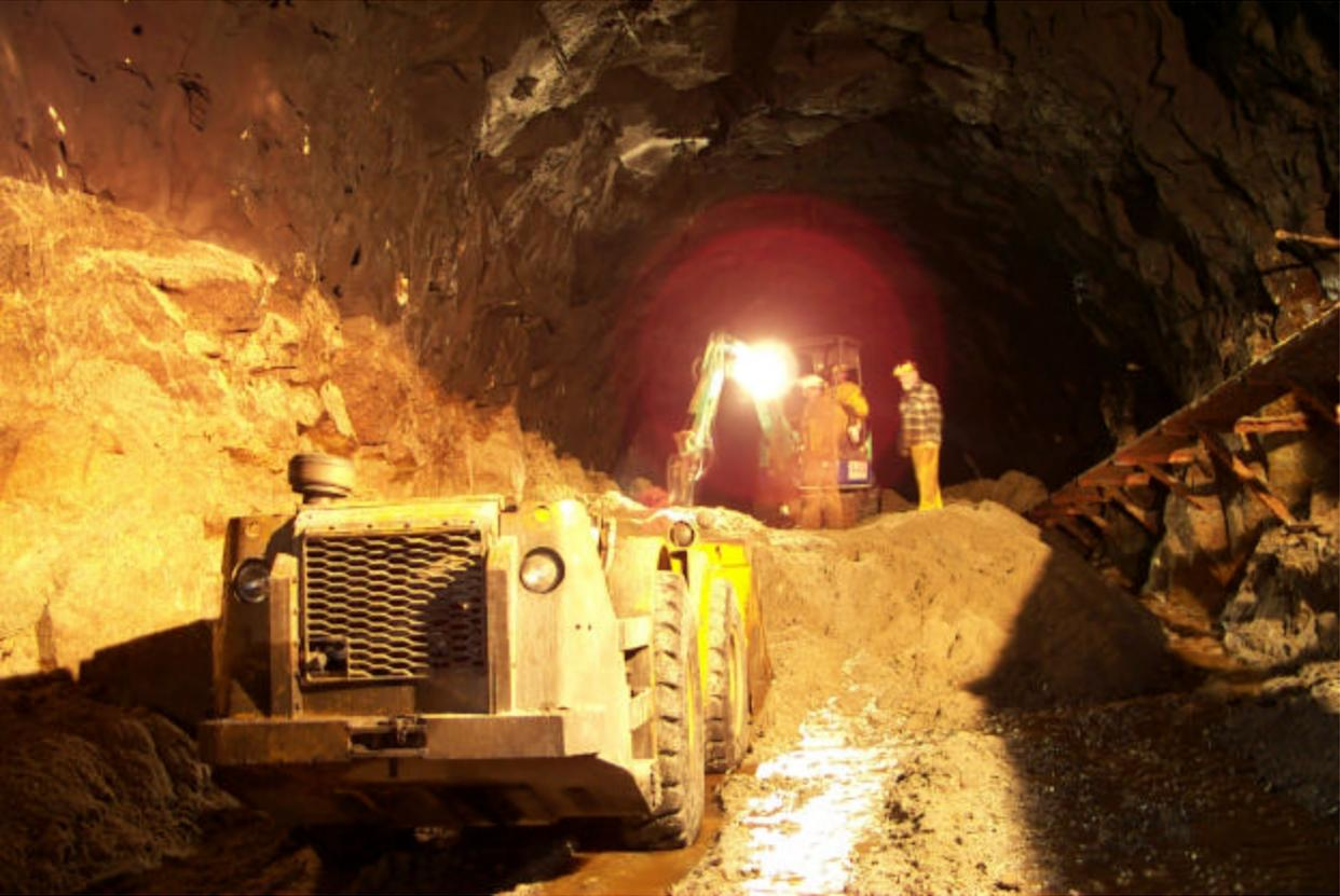
**Cleaning end of Rock Trap. Note discoloration line showing filled area of trap.**
