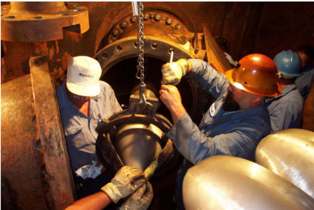
Installation of prototype nozzle seat ring and needle tip
