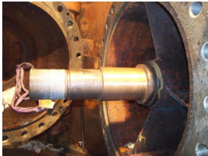
**Existing housing and guide vanes. Note: Poor existing surface finishes**
